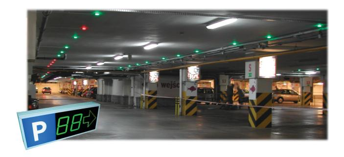
Parking Guidance System based on single space sensors for underground and multi storey car parks.
