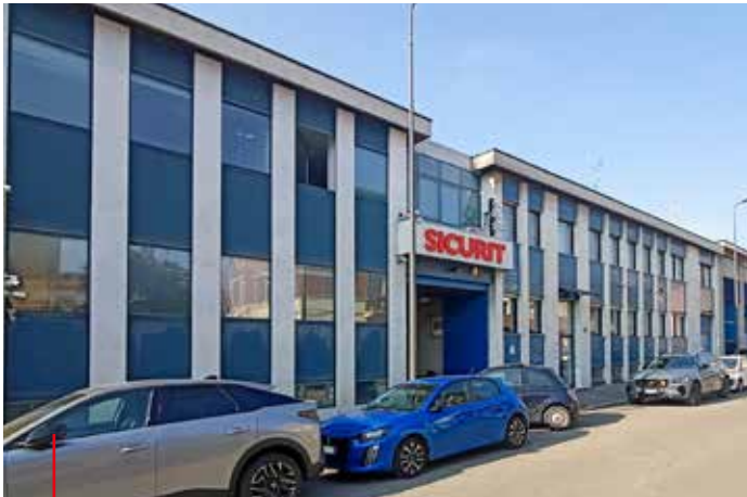
Milan HQ offices
